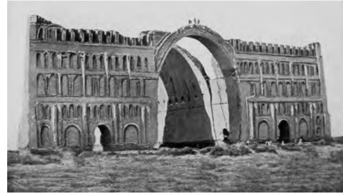
Fig. 91: Ctesiphon, Sasanian Palace from the time of Khosrow I, 531–579 A.D. (condition before 1888). The facade of the Ctesiphon Palace shows a giant iwan, the Taq-i Kisra (the arch of Khosrow) in the centre, flanked on each side by rows of blind niches in five stacked registers. (The ensi shows a comparable composition in the fields with the gush motif and the niche. Cf. fig. 97). This form of a barrel-vaulted iwan as a throne and audience hall goes back to the Parthians (an early form is the iwan of Mansur-Depe near Nisa. See Ellerbock/Winckelmann 2012: 88). It found its continuation and wide distribution in Sasanian and later in Islamic art. Repr. from Erdmann 1943 (1969): Plate 5.
